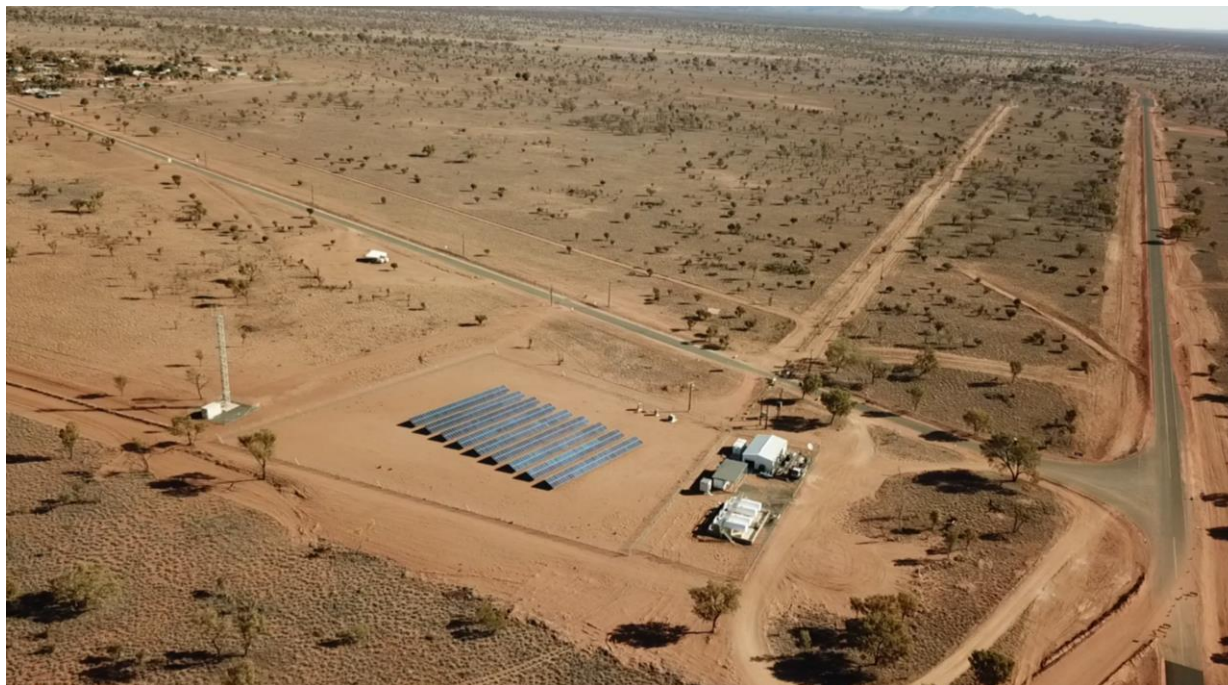
Photo 1: The Community of Atitjere can be seen in the top left hand. Mica Road runs diagonally toward the bottom right hand of the photo. The Plenty Highway is seen running down the right hand side of the photo. The commencement of the bypass can be seen just below the intersection.
