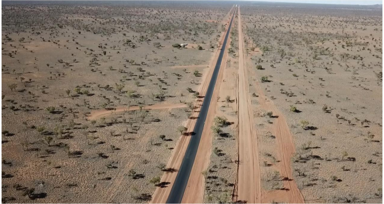
Photo 2: Heading east, the new bitumen on the plenty Highway and running parallel to it, the unsealed bypass road.
