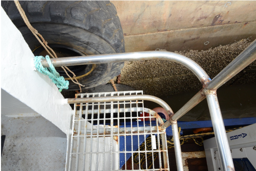
Photo 5 showing edge of protruding bridge wing
