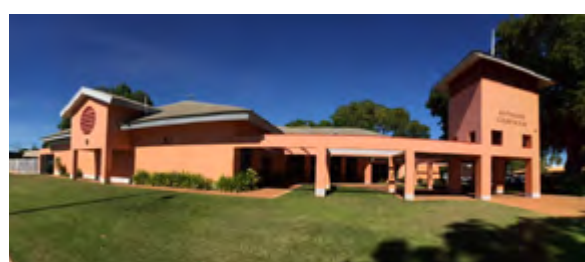
The new wing at the Katherine Courthouse.
